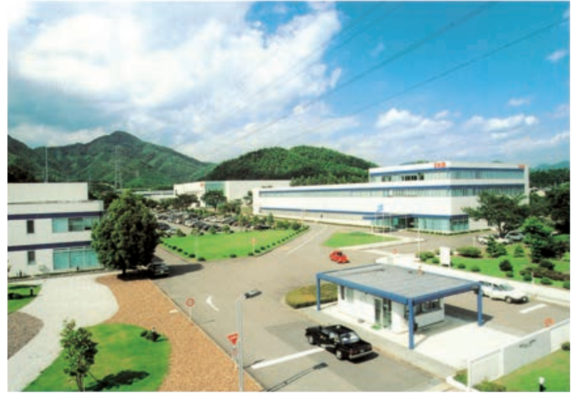
Gifu factory main entrance
